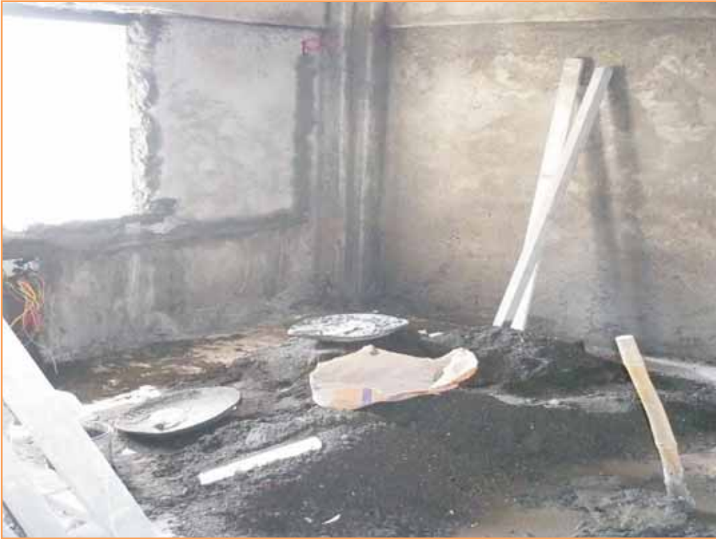
2nd Bedroom Plastering Work
