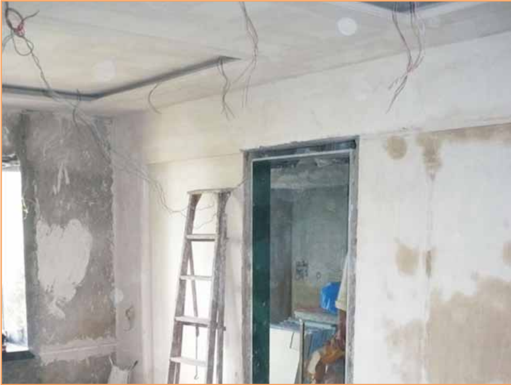
Living Room pop Walls and Ceiling Works
