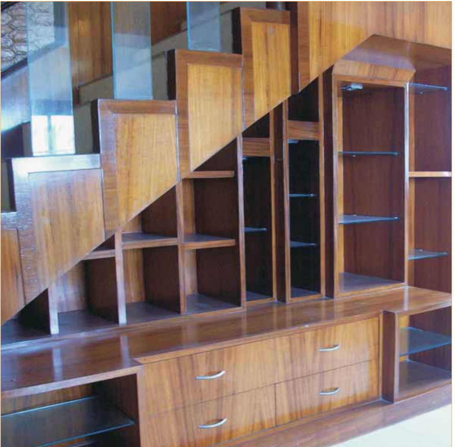
Staircase with storage with display below
