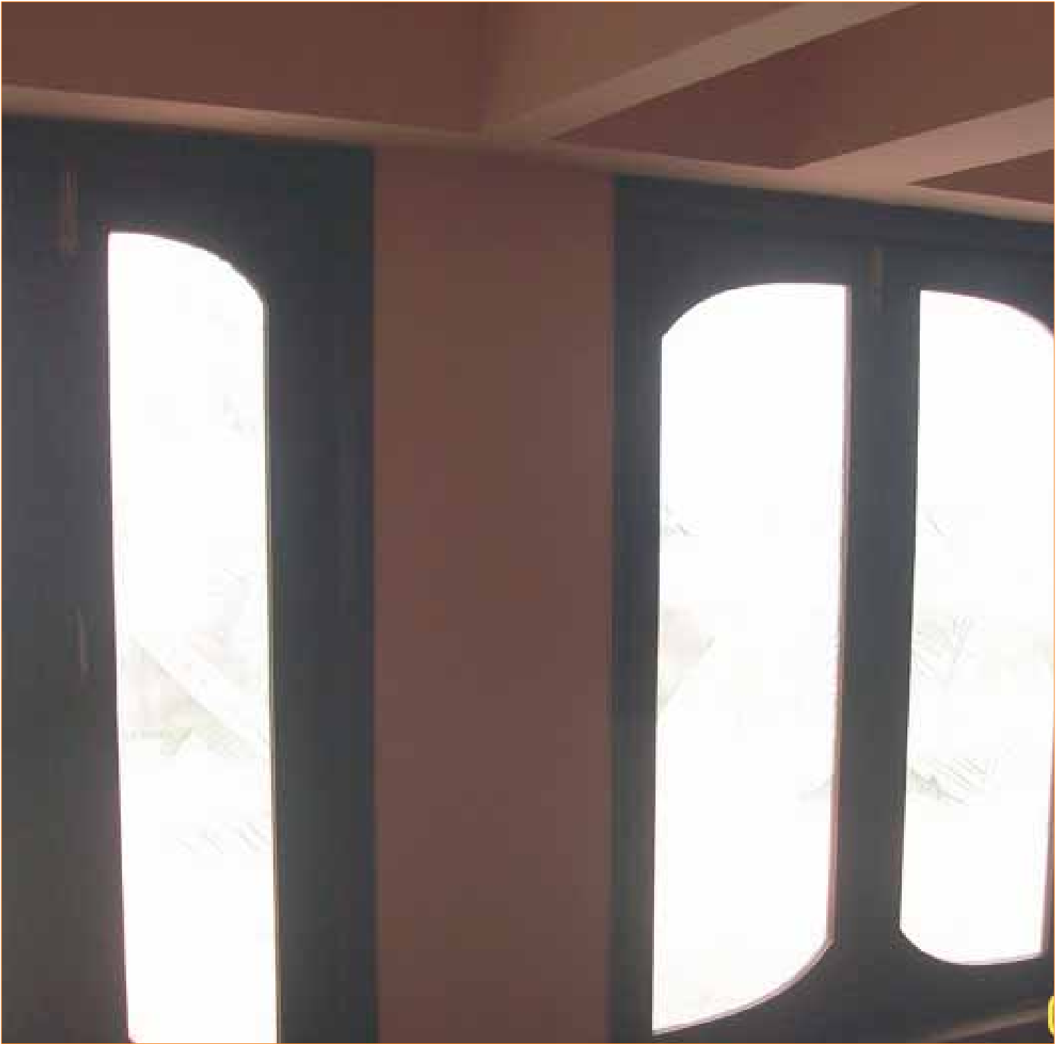
Windows with false ceiling
